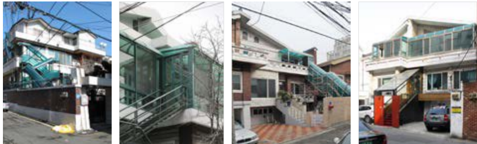
Modified houses: balconies are converted and and stairs added, car parkings replace gardens and walls and gates.
