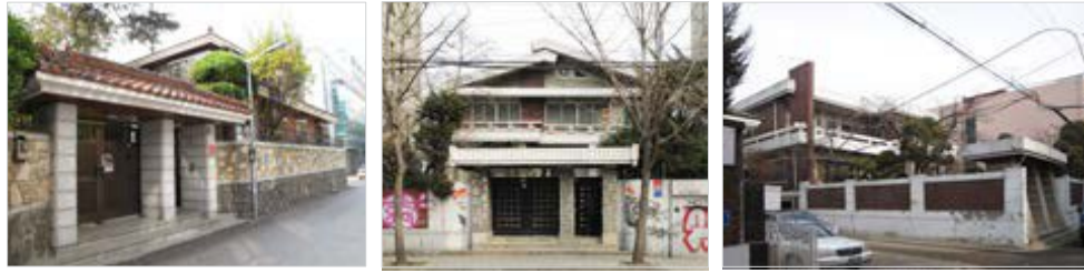
Original houses, typically with garden, wall and gate
